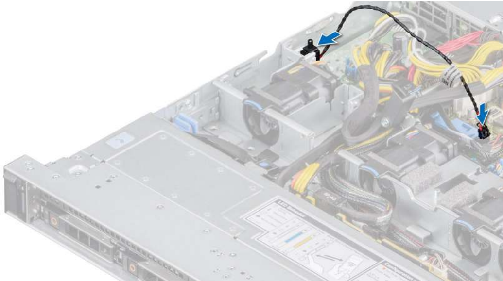
Figure 26. Installing the intrusion switch
