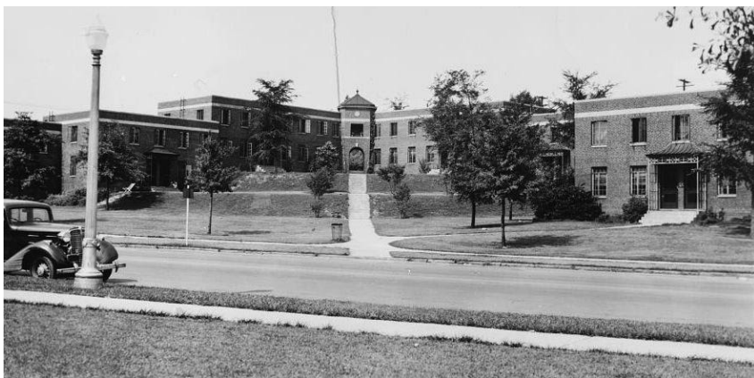
Figure 4-6. Techwood housing project Atlanta, Georgia. America's first federally funded low-income housing. Shown in late 1930s. Largely demolished 1999. Image: Wikimedia commons.
