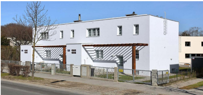
Figure 5-5. The semi-detached house Jagdschloßgasse 80, 82 of the Werkbundsiedlung Vienna in the 13th district of Hietzing. Semi-detached house built around 1930 according to plans by the architect Arthur Grünberger. It is part of a model estate of around 70 houses with around 50 different house types that were built between 1929 and 1932. More than 30 architects took part in the planning of the individual houses. Image: Bwag, Wikimedia Commons.
