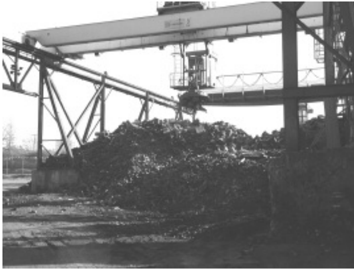
Figure 2—The Raw Materials Storage Yard of the Foundry.
