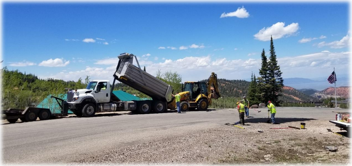
Asphalt Repair Inside Radius
