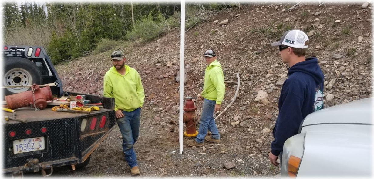
Hydrant Repair on top of Steam Engine (Rex, Jason, Kade)
