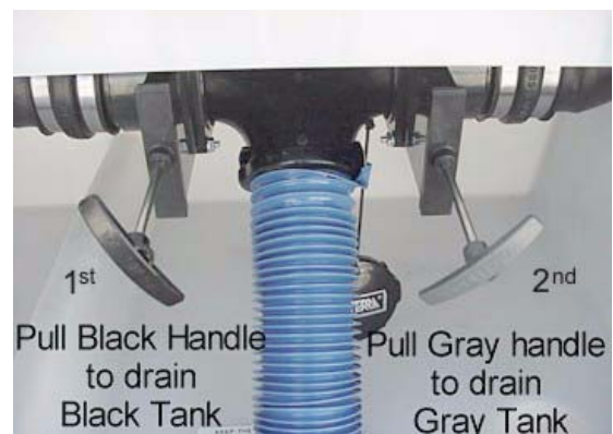
Holding Tank Valves (Typical)
