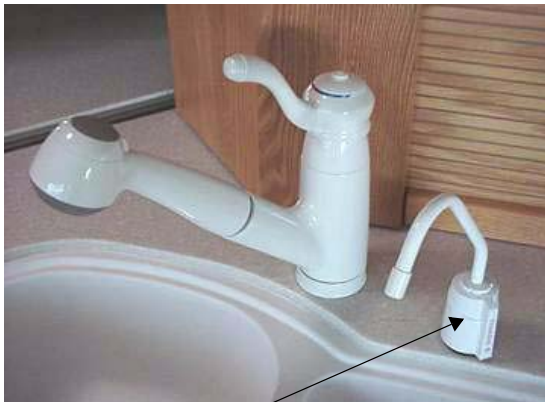
Filtered Water Faucet (Typical)
