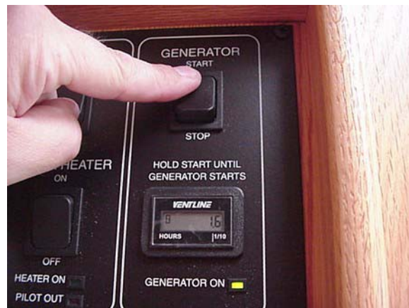
Generator Switch and Hourmeter
