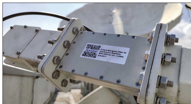
Figure 6. C-Band BPF Inserted into Feed Network
