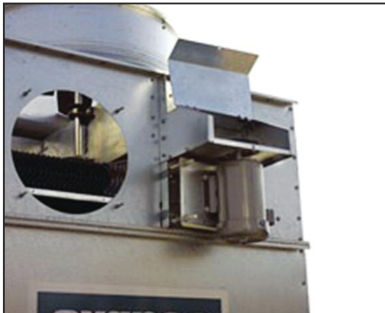
External Motor Mount (with swing away cover)
