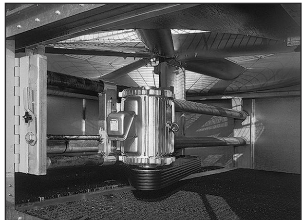
Motor Base Assembly
