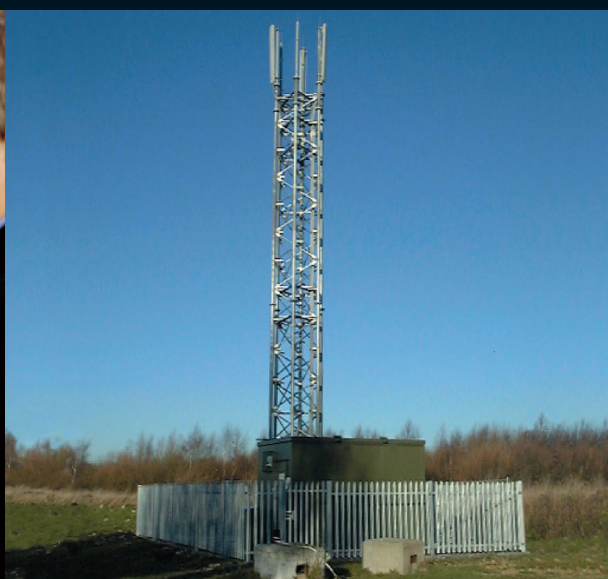
Base station showing antenna, lattice mast and cabinet
