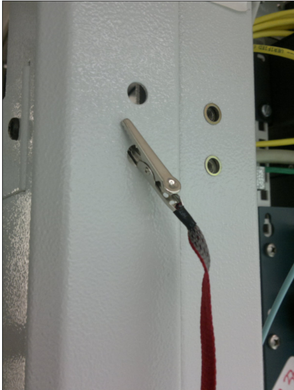
Figure 2-21 Temporary Wrist Strap Connected to a Non-conductive Part of the Rack
