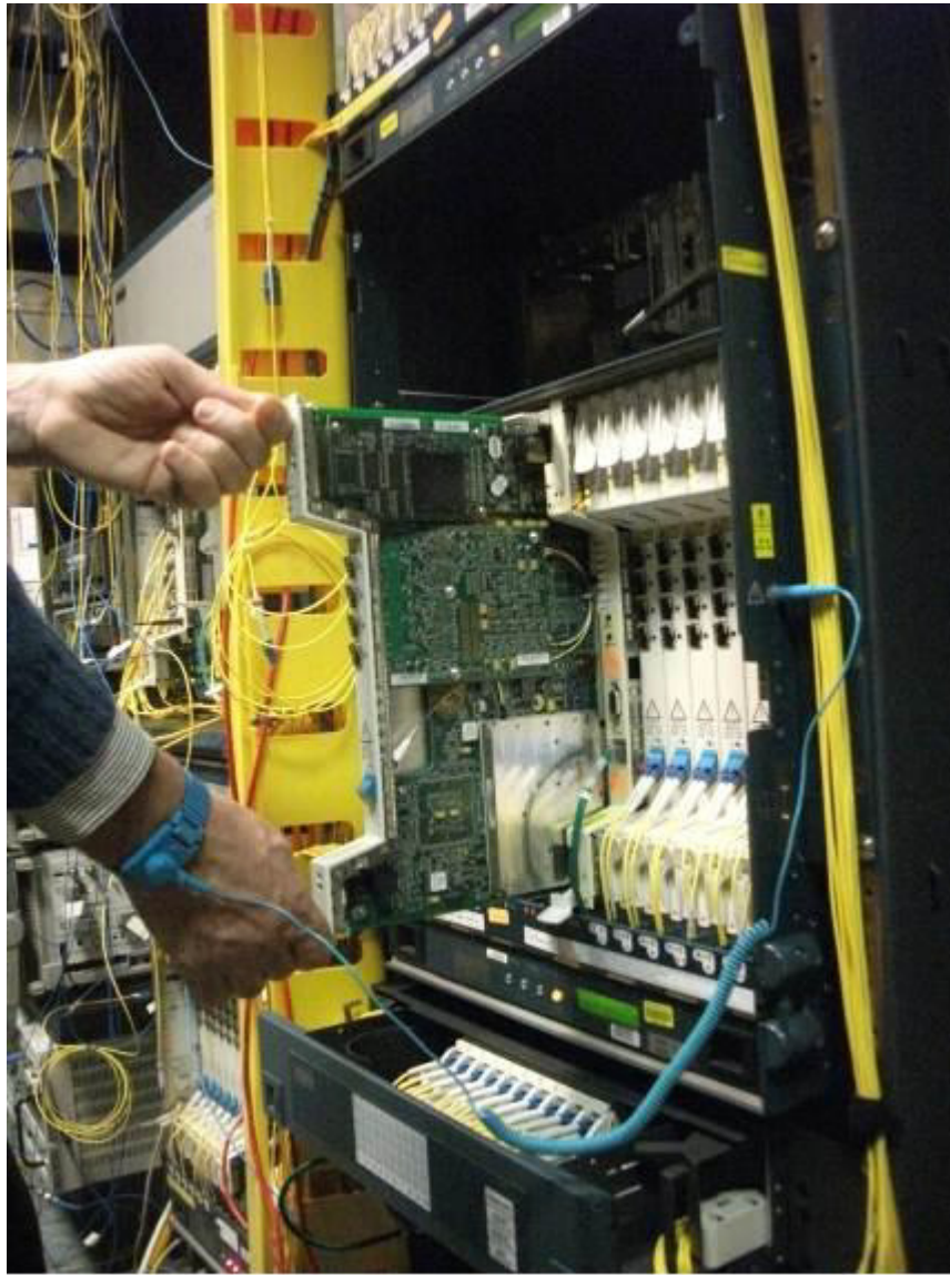
Figure 2-23 How to Handle Cards during Installation
