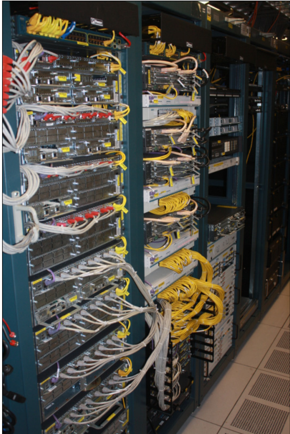
Figure 2-4 Proper Cabling
