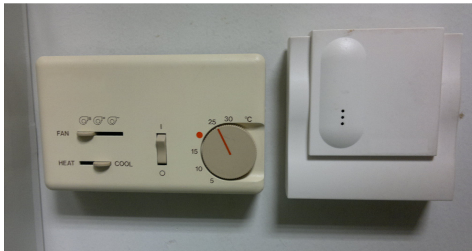
Figure 3-22 Temperature Monitoring Devices
