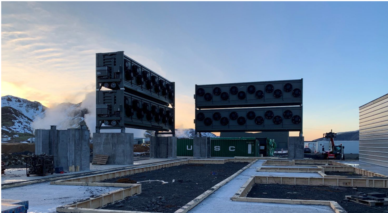
Under construction: Climeworks' new large-scale direct air capture and storage plant "Orca" (Credit: Climeworks)
