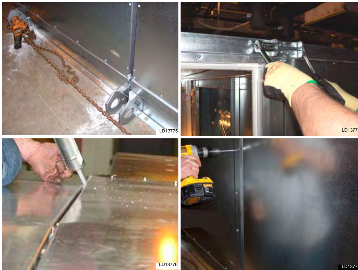
FIG. 2-20 – BRINGING SECTIONS TOGETHER
