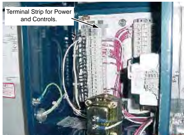
FIG. 2-57 – MAIN POWER AND CONTROL PANEL W/ COVER OPEN
