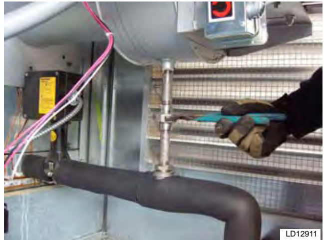
FIG. 3-20 – CONDENSATE DRAIN
