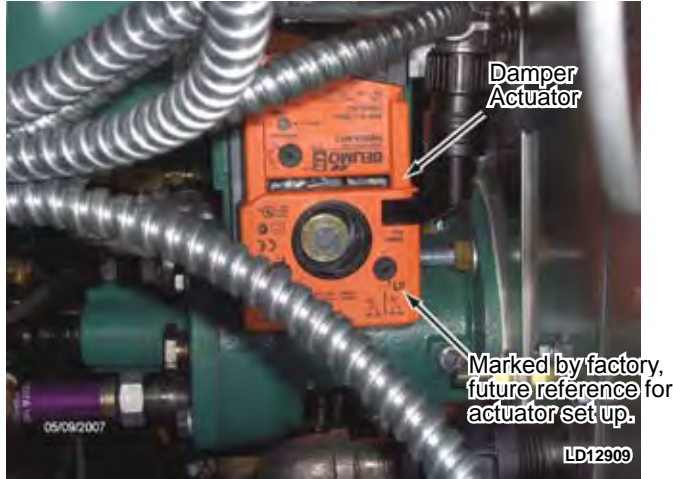
FIG. 3-19 – DAMPER ACTUATOR
