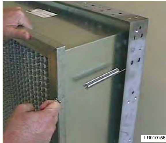
FIG. 2-111 – FRAME WITH 4 LATCHES INSTALLED
