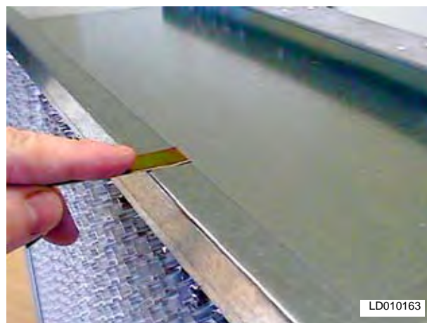
FIG. 2-112 – PREFILTER LATCH AFTER INSTALLATION ONTO FILTER HEADER.
