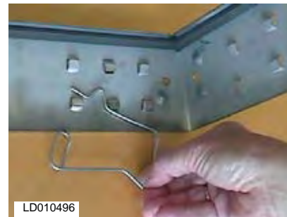
FIG. 2-104 – INSTALL LATCH P//N 026-35778-007
