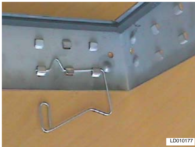
FIG. 2-101 – CORRECTLY INSTALLED LATCH P/N 026-35778-007
