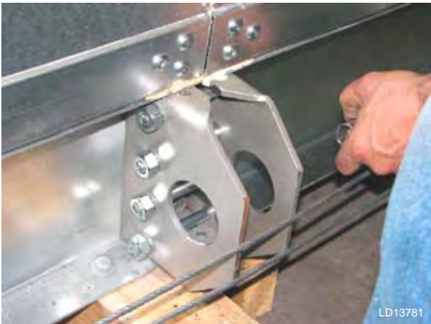
FIG. 2-28 – INSTALLING BOLTS AFTER PULLING UNITS TIGHT TOGETHER
