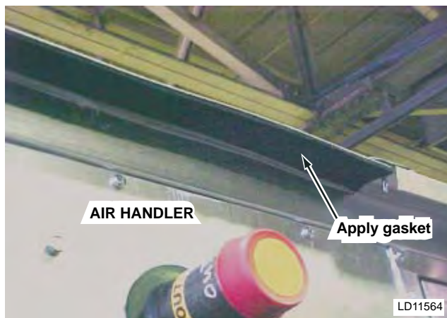
FIG. 2-41 – INSTALL GASKET UNDER ROOF OVERHANG
