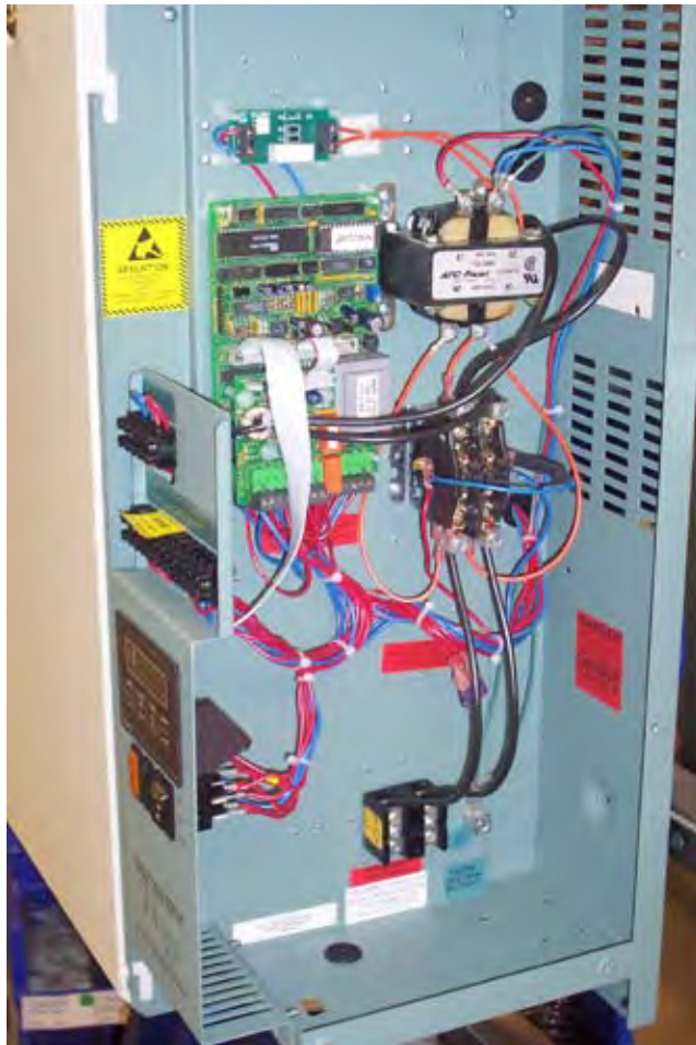
FIG. 2-62 – TYPICAL HUMIDIFIER PANEL LAYOUT
