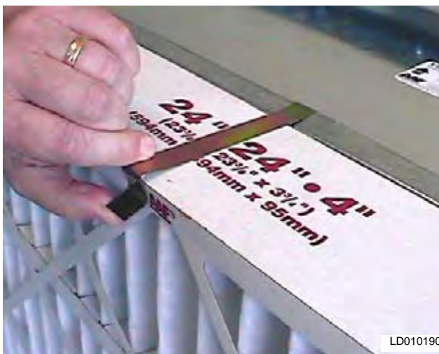
FIG. 2-114 – SPRING THE END OF THE LATCH SO THAT IT FITS OVER THE EDGE OF THE PREFILTER. (4" W/026-36339-000 LATCH SHOWN)
