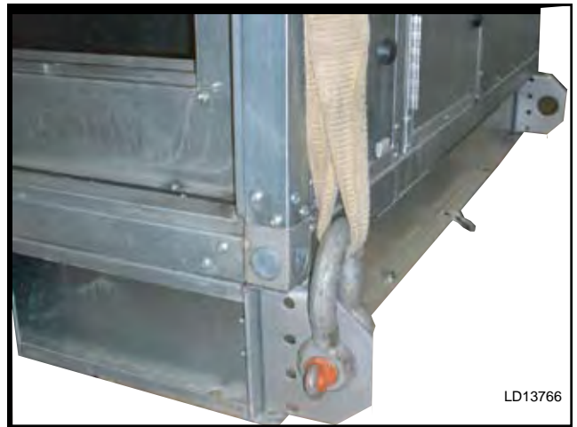
FIG. 1-6 – RECOMMENDED LIFTING WITH BASERAIL
