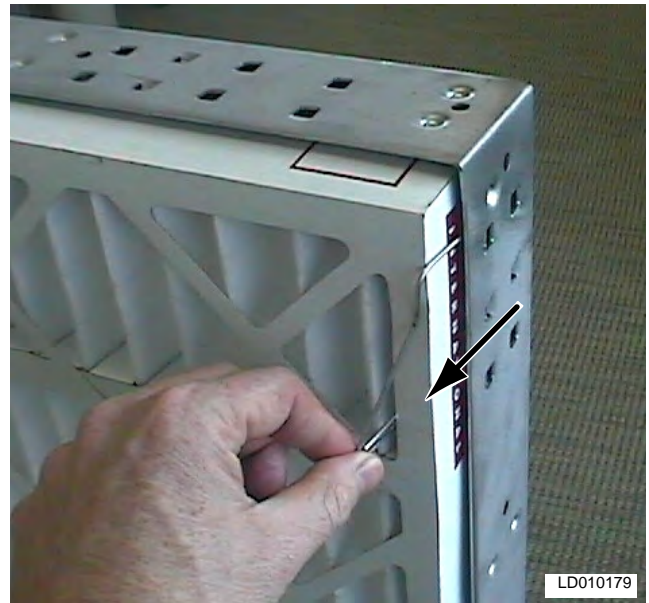
FIG. 2-102 – PLACE THE END OF THE LATCH OVER THE FILTER FRAME, SECURING THE FILTER TO THE FRAME.
