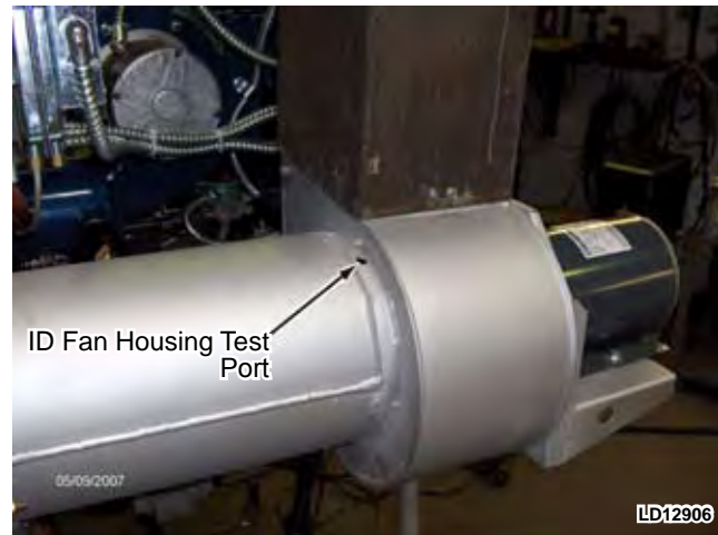
FIG. 3-18 – FLUE (STACK) COMBUSTION TEMPERATURE AND EFFICIENCY TEST PORT
