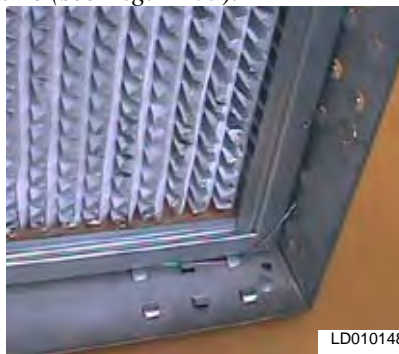
FIG. 2-103 – INSTALLED CARTRIDGE FILTER
