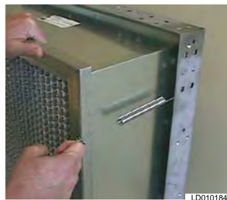
FIG. 2-109 – SPRING LATCH SHOULD BE PULLED AND FASTENED IN HOLE IN THE HEADER OF THE FILTER.
