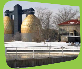
Back River Wastewater Treatment Plant in Baltimore, MD
