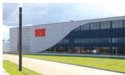
Plant for large gear units, Bruchsal, Germany
