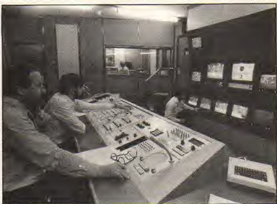
Production control room for the larger of the two studios, Studio 1. Through the window in the background can be seen the sound control room.
