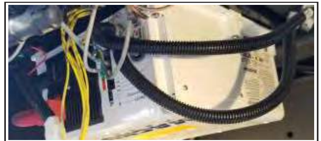
Figure 10-11: Converter/inverter
