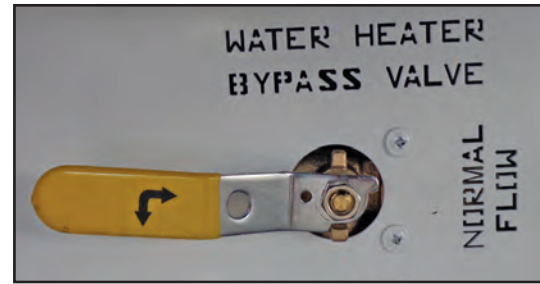
Figure 14-8: Water heater bypass valve
