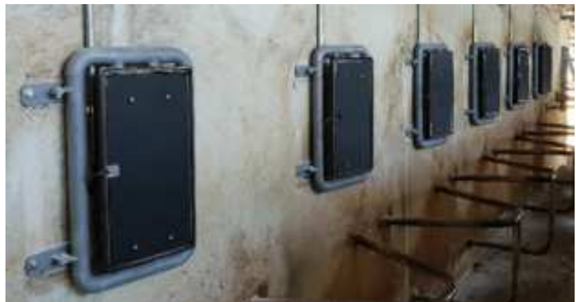
Herringbone Parlor – 50 cm antenna mounted on the wall.
