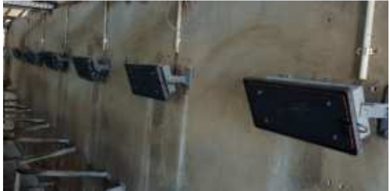
Herringbone Parlor – 40 cm antenna mounted on the wall.
