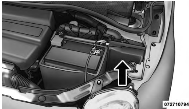
Front Distribution Unit
