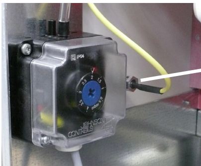
Cooling air pressure switch
