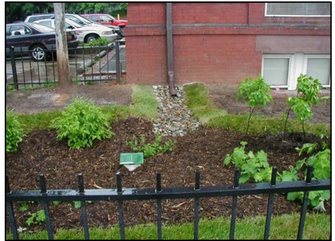
Rooftop disconnection. Source: LID Center
