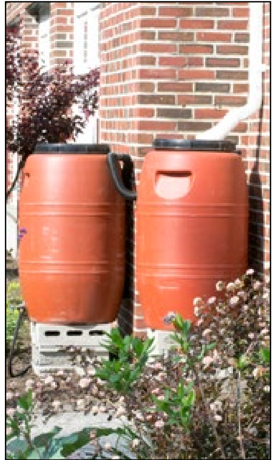
Photo Source: City of Portland
