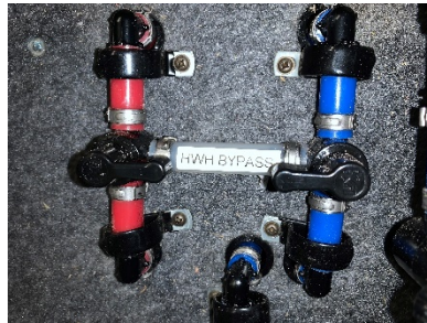
HOT WATER HEATER BYPASS
