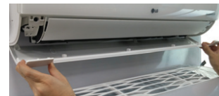
Figure 76: Checking that All Attachment Locations Are Secure (Step 5).
