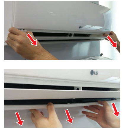
Figure 46: Removing the Bottom Cover, Alternate View.
