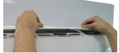
Figure 77: Disassembling the Air Filter (Appearances May Vary Depending on Indoor Unit Model).
