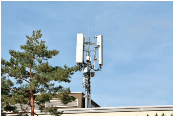
Huawei’s Super BladeSite solution is commercially available. The solution features a component-based design for blade RRUs, BBUs, power systems, batteries, and microwave. It is a full outdoor site solution that does not require an equipment room or even cabinets. One simplified site can accommodate 2G, 3G, 4G, and 5G, allowing for easy, flexible deployment and enabling carriers to scale up 5G rollout faster.
