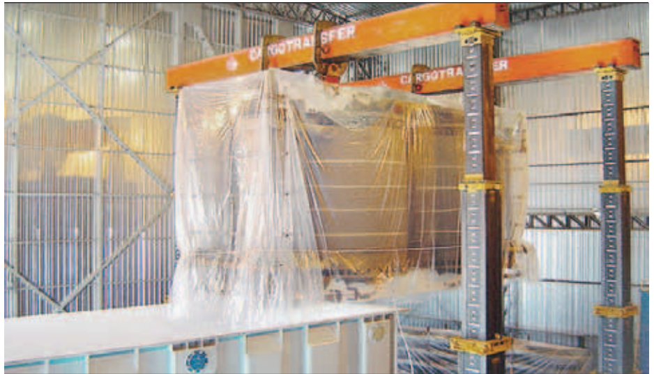
2 Untanking at site of a 440 MVA/550 kV transformer to replace windings
