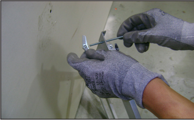
Figure 4.5 Toggle Bolt Installation through Mounting Bracket
