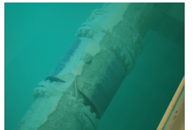
Submerged Water Treatment Plant
