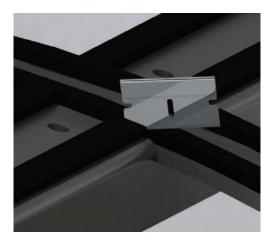
Figure 45. Cutting gasket for tight joints
