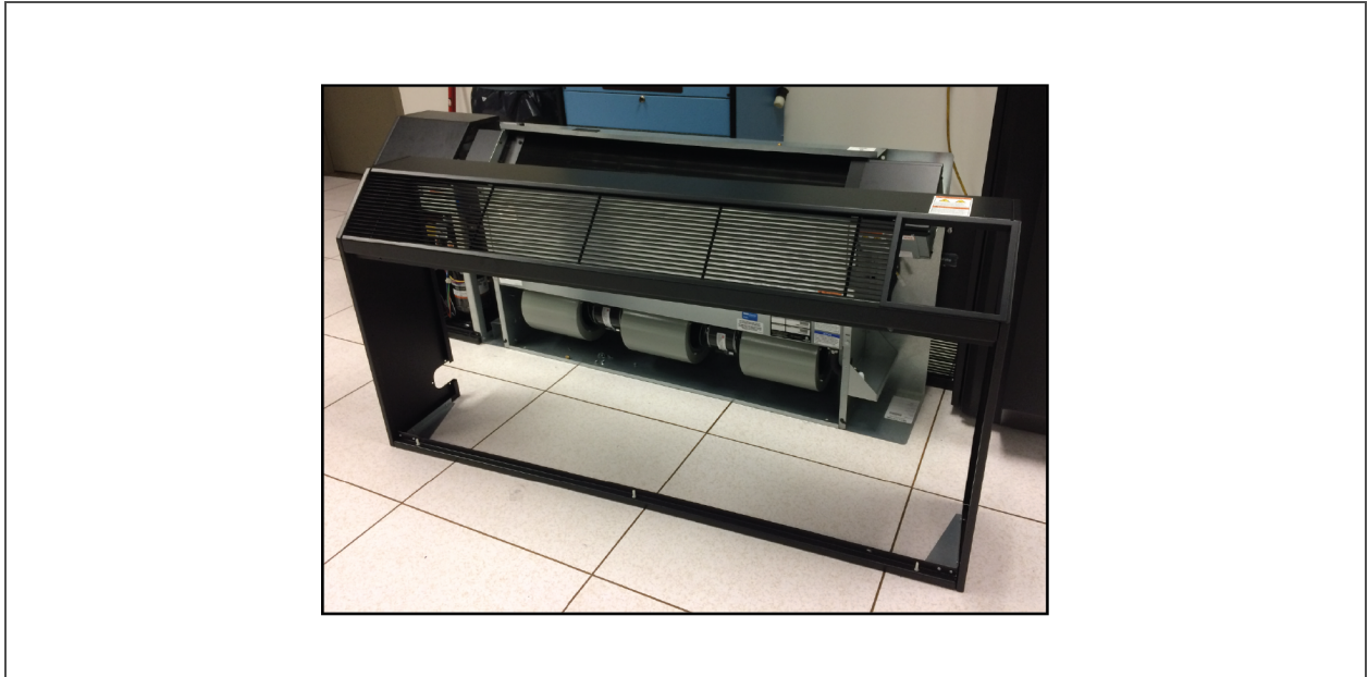
Figure 4.3 Remove Evaporator Panel Assembly
