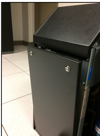
Figure 4.7 Remove Front Access Panel from Condensing Unit
