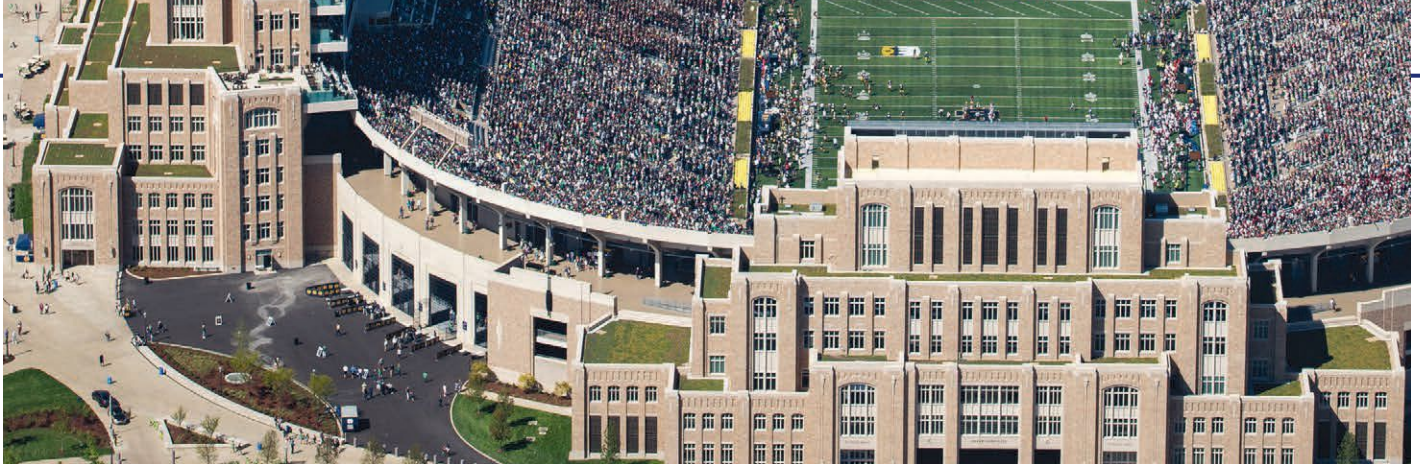
GREEN ROOFS ADORN THE NEW BUILDINGS THAT ARE ANCHORED TO THE SOUTH, EAST AND WEST SIDES OF THE STADIUM.
