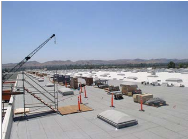
Exhibit 1. The rooftop looking south.
