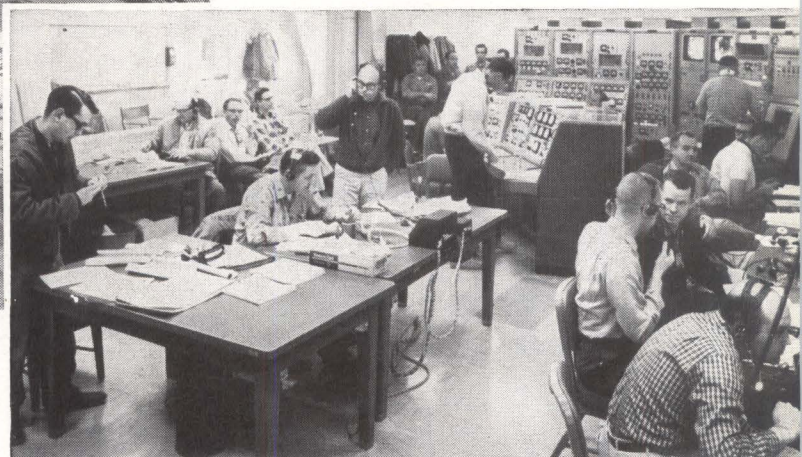
CONTROL POINT for remote operation of Kiwi reactors during tests
