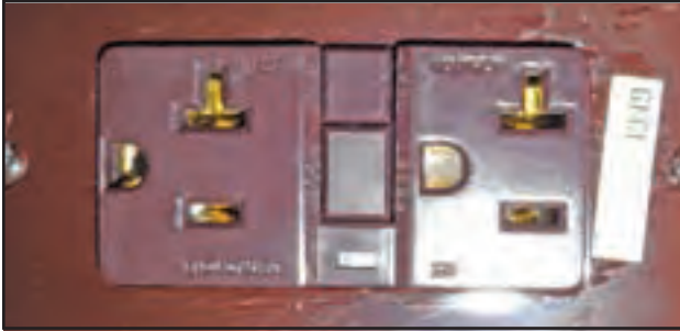
Figure 9-10: GFCI receptacle
