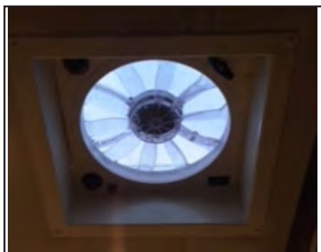
Figure 14-3: Overhead vent fan
