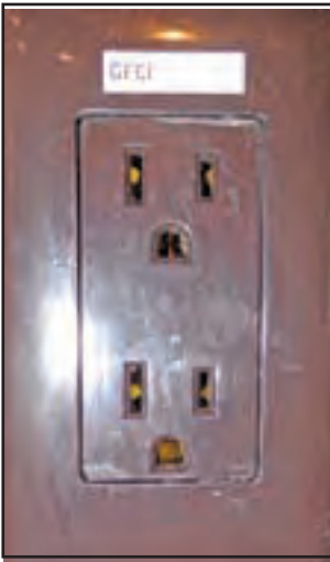
Figure 9-8: 12 VAC receptacle
