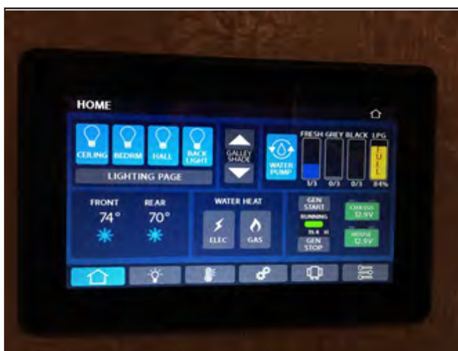
Figure 5-7: Water heater controls
