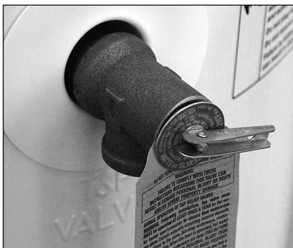
Figure 25 - Temperature and Pressure Relief Valve
