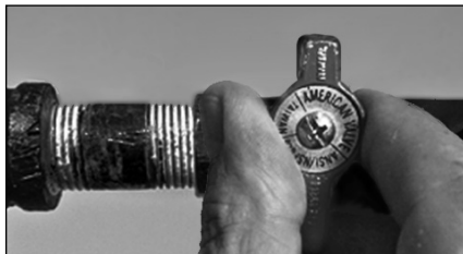
Figure 50 - Gas valve in “off” position.
