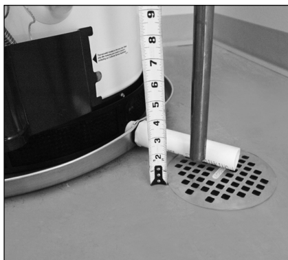
Figure 26 - Temperature and Pressure Relief Valve Pipe
