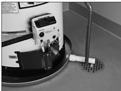
Figure 23 - Metal drain pan piped to drain.
