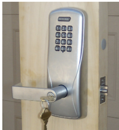
Finished CO Lock Install Front View
