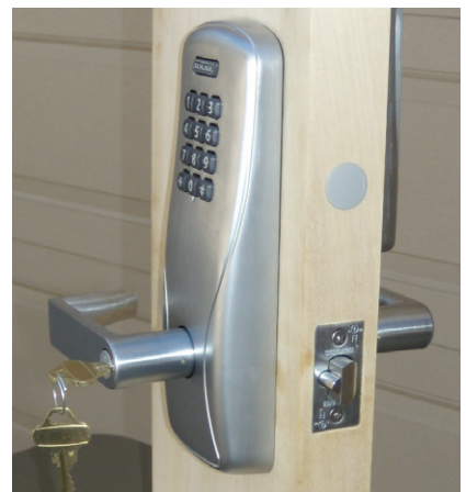
Finished CO Lock Install Edge View
