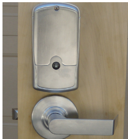
Finished CO Lock Install Rear View
