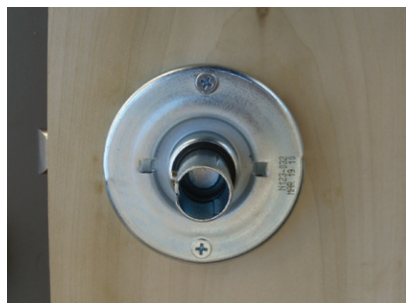
Installed Spring Cage with Inside Spindle
