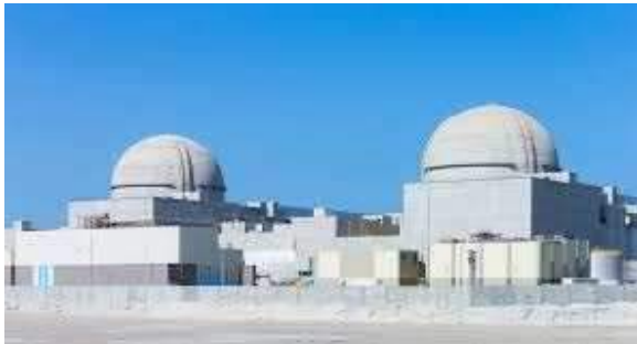
Barakah new build in UAE
