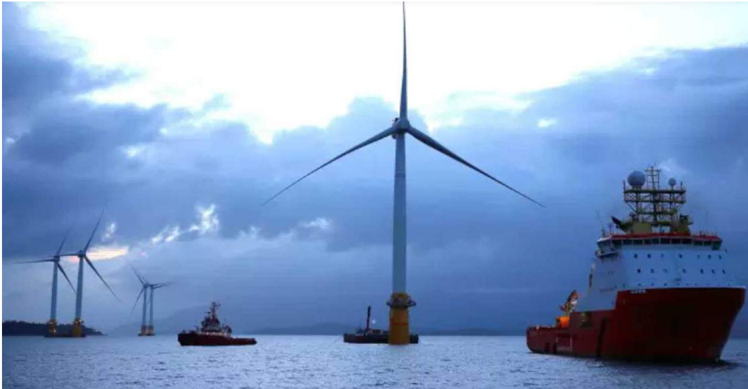
5 x 6MW Floating Spars installed in 2017 off Peterhead (Courtesy Equinor)
