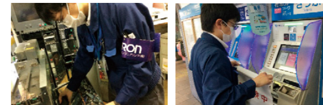
Maintenance work at station halls
