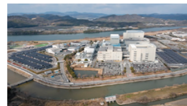
Left: No.1 Solar Power Plant Right: No.2 Solar Power Plant
