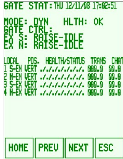
Figure 3-7 Typical Gate Status Display
