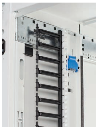
Medium-duty vertical cable manager
