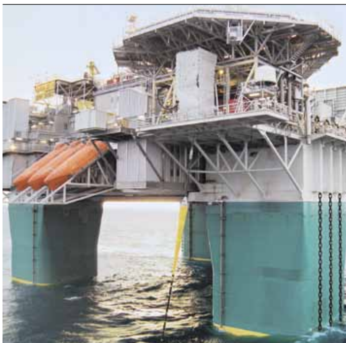
9 The Gjøa platform with the cable being pulled aboard.
