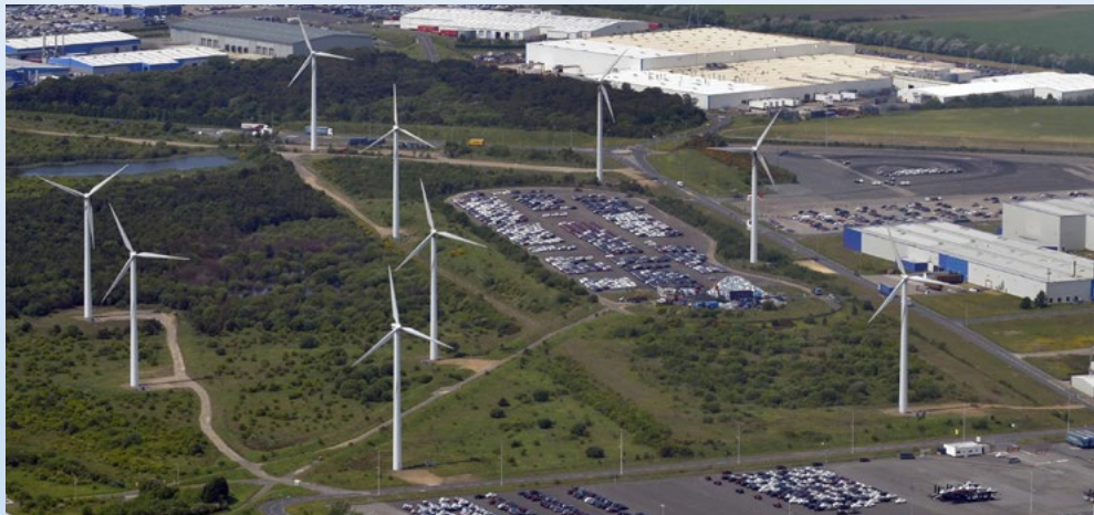
Power-generating wind turbines at Nissan Motor Manufacturing (U.K.).
