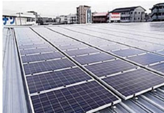
Solar panels are on the roofs of some Kanagawa Nissan dealerships. Power from the panels is supplied to dealerships through the PPS system.
