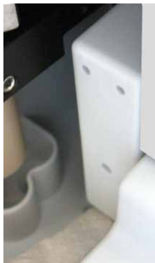
Fig. 42: Drying the leak sensor
