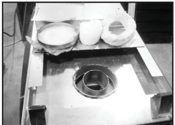
Figure 9.5 Remove and discard the seal cap, insulation donut, insulation plug, and the insulation basket. Attach the first vent section (it will snap into place). Slide the vent gasket onto the vent section and then, up against the appliance. Secure the vent gasket to the appliance with two self-tapping screws found in the manual bag. Note: The vent gasket can found in the manual bag.
