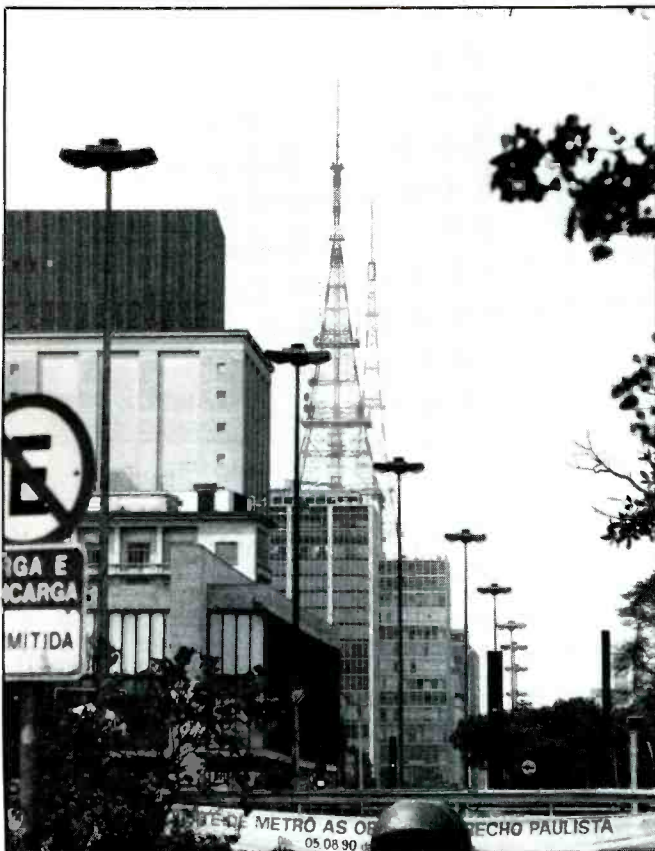
Two broadcast towers on the main drag in Sao Paulo, Brazil. The first tower is used by TV Channels 5 and 11. The second tower is used by TV Channel 16. Thanks to Helio Soares, Sao Paulo, Brazil, for the photo.
