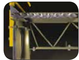
Truss Girder & Bar Joist
