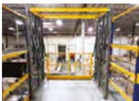
Pallet Drop Zone Gate
