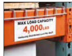
T4: Beam Load Capacity Label
