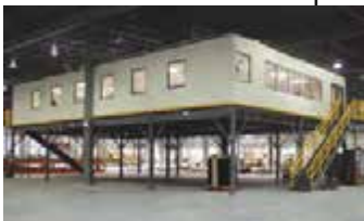
Offices on Pre-Engineered Mezzanine
