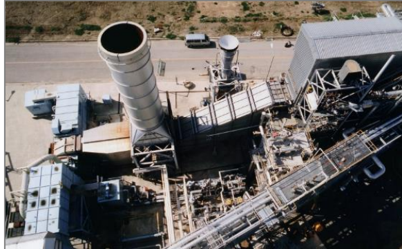
20+ years of operation 6B operating on high H 2 ( 70-95% H2 ) with more than 180k hours
