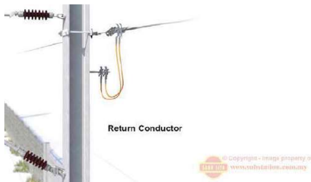
Return Conductor using Double Short Rail Earth
