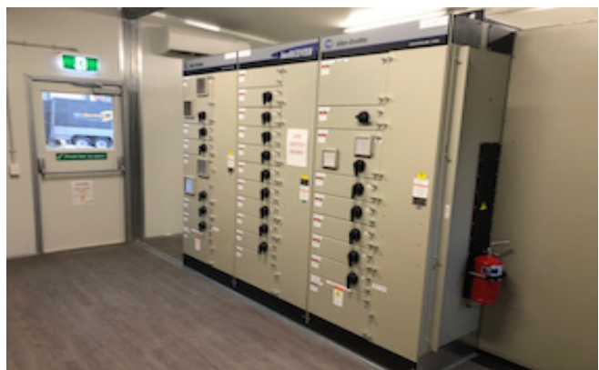
The new smart motor control solution which provides key diagnostic information that optimises performance with real time access to operation and performance trends
