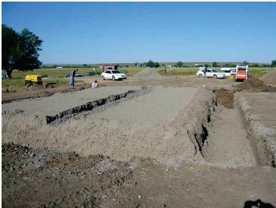
Figure 9. Over-Excavated, Compacted, Filled, and Shaped Subfoundation
