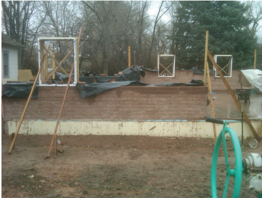
Figure 10. Window Bucks Installed
