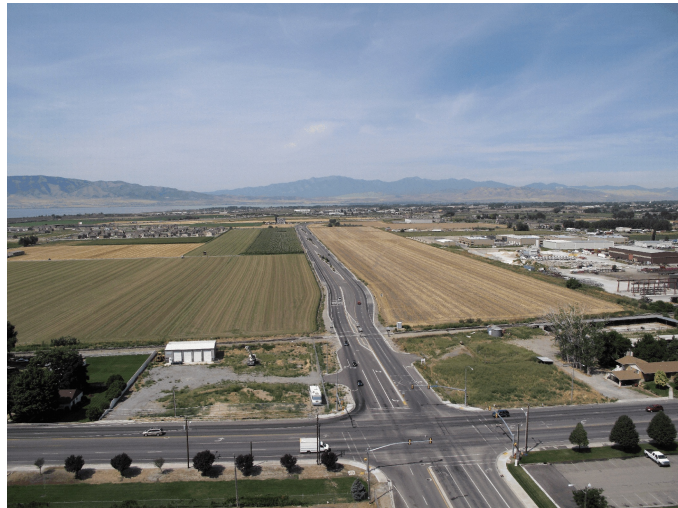
700 North Corridor, west of Geneva Road
