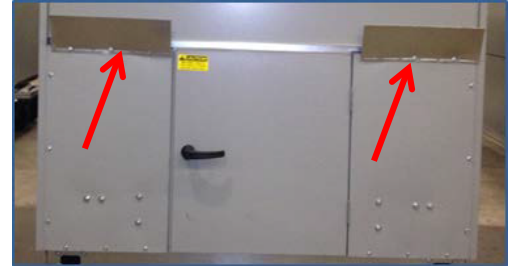
Figure 13: Remove and Discard the Shipping Foam (Step 3).
