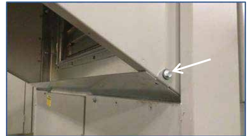
Figure 28: Location of Top Filter Rail (Step 4A).
