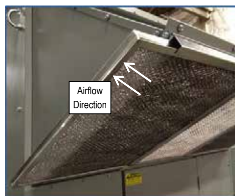
Figure 30: Install Filters with Arrow Pointing Into the Unit (Step 5).
