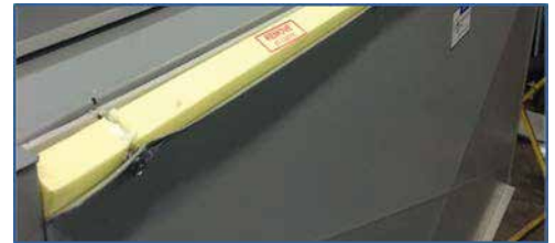
Figure 13: Remove and Discard the Shipping Foam (Step 3).
