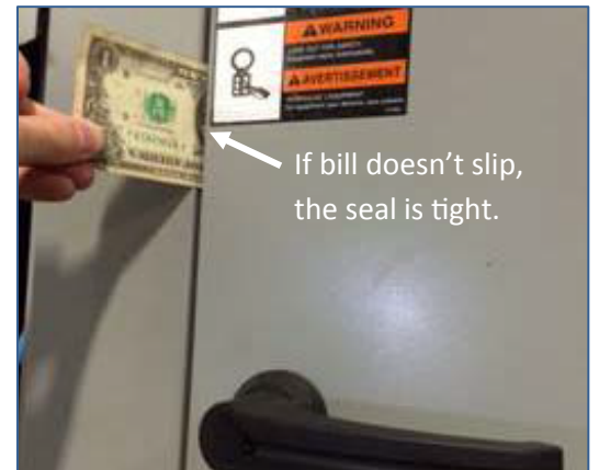
Figure 94: Checking the Access Door Seals.
