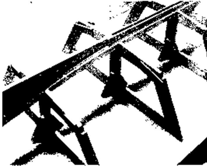
KEELSON & STEM SET UP OVER THE MOULDS. NOTE CLINCHBOARD SCARF AND RABBET FOR BOTTOM PLANK.
